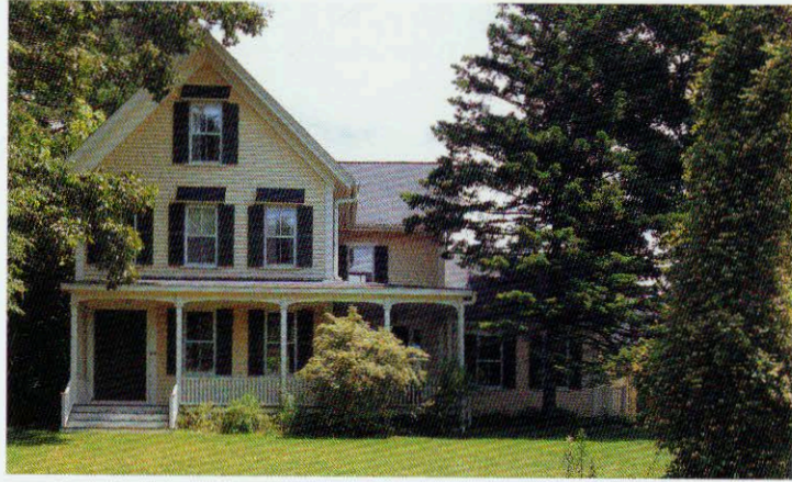
◀▼ The back of the house (below), which was not subject to such rigorous historic review, contrasts dramatically with the more formal and classic front (left). Pastel-colored stucco panels on the main house are repeated on the studio addition, which is connected to the house by a pergola-covered walkway.
